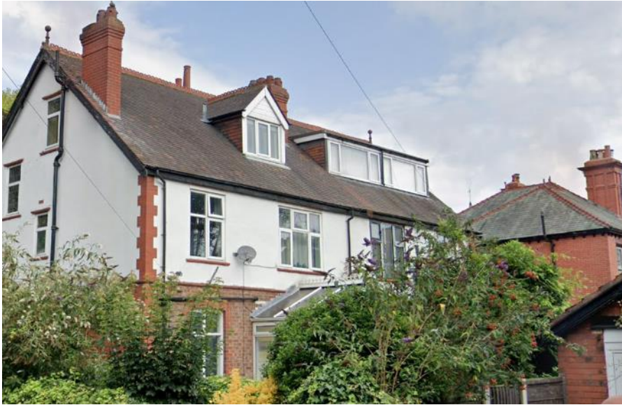
Rear elevation of 91 Palatine Road (R/h side) with No.93 on the left, from Danesmoor Road
