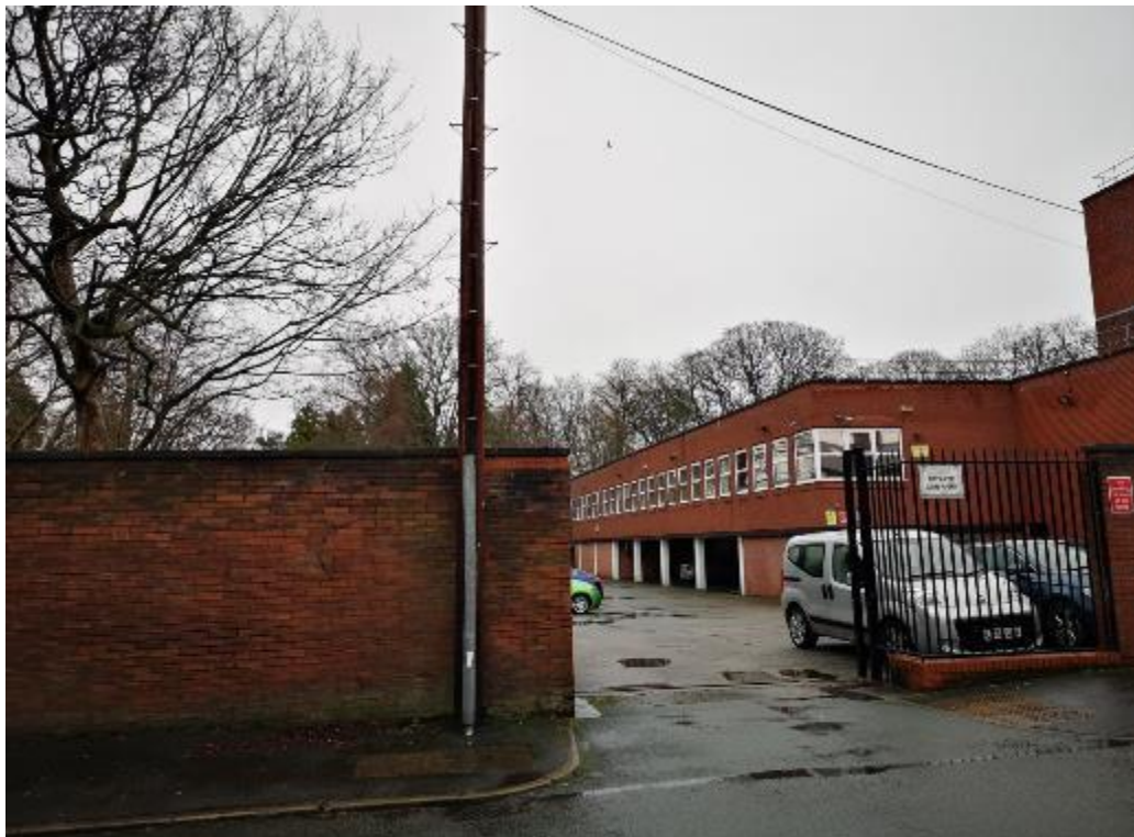
Rear of Usdaw offices as viewed from Langley Road
