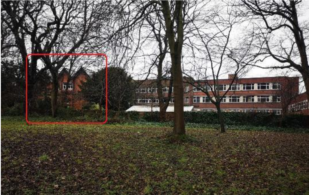
View south from Platt Fields Park towards the application site the original Villa to the left highlighted in the red box and later three storey extensions to the right
